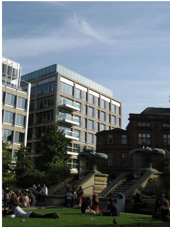
Case Study Building
